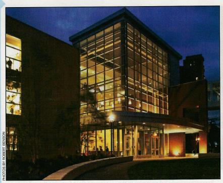
Red and buff brick lend a warm tone to the building's exterior, while clear- and fritted-glass curtainwalls trimmed in aluminum allow the facility to serve as a beacon of activity.
